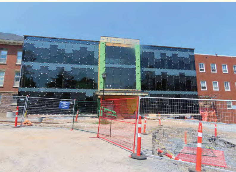
Engineering Commons under Construction.
