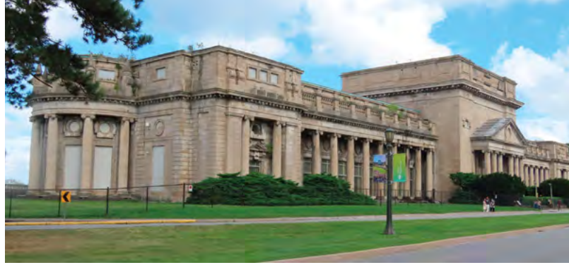
Toronto Power Generating Station, in 2024 Photo by Pat Brennan.
