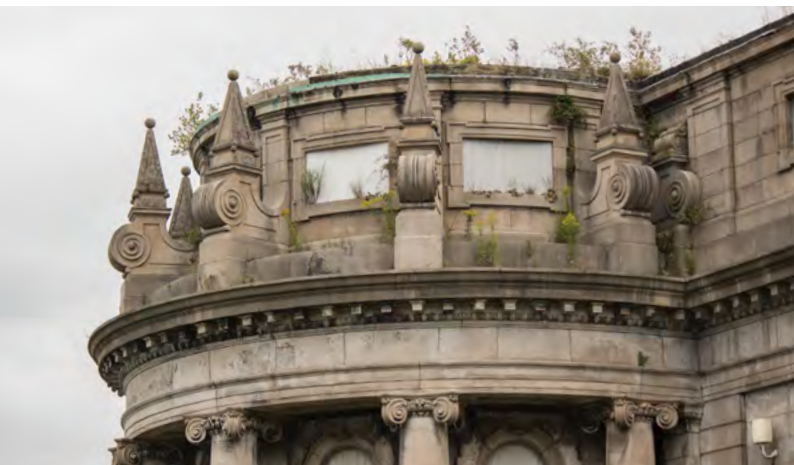
Toronto Power Generating Station on Aug 29 2024. Photos By Benito Del Monte.
