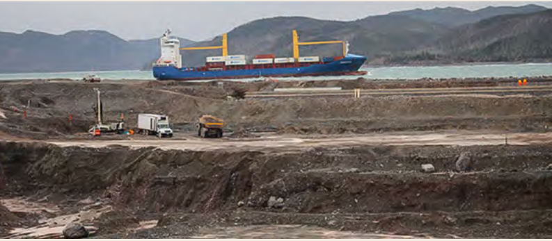
Argentia - graving dock. Photo courtesy of Cenovus Energy.
