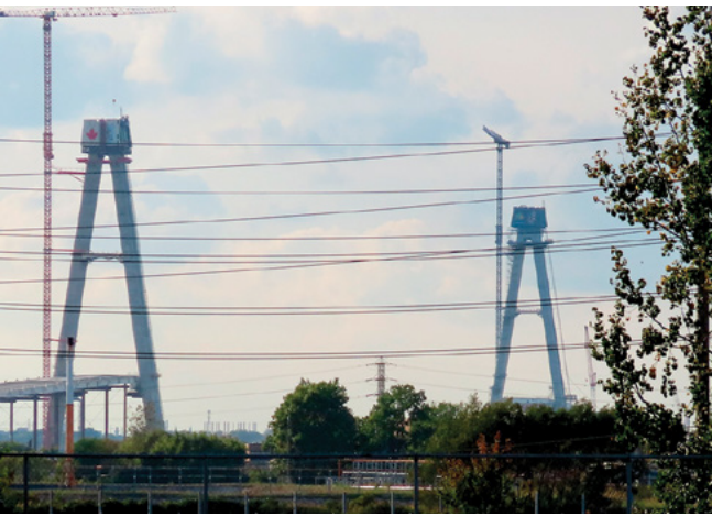
72-storey tall concrete towers on both sides of the Detroit River that will hold the steel cables that will support the 7,200-foot-long bridge deck. Photo By Pat Brennan.
