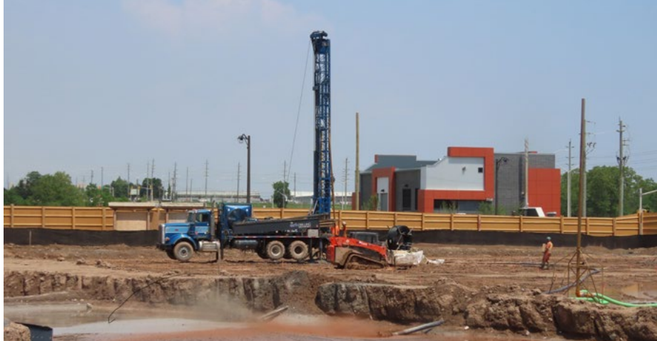
STS Geothermal drilling for Mattamy Homes.
