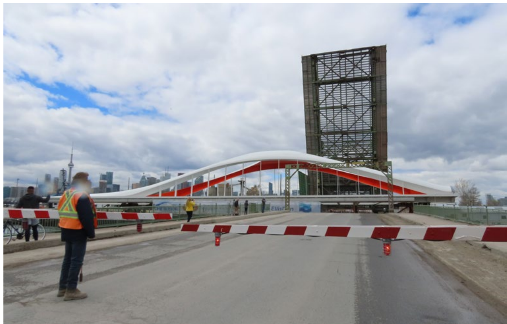
2nd bridge under Cherry Street waiting to be installed in place.
