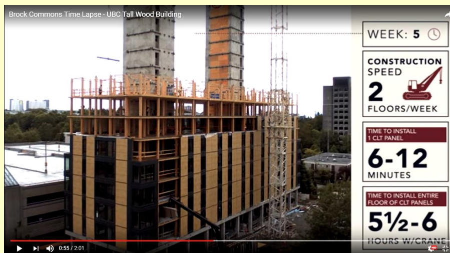
Two minute time lapse video shows Brock Commons' 17-storey tall wood installation, completed in 9½ weeks. See https://www.youtube.com/watch?v=GHTdnY_gnmE
