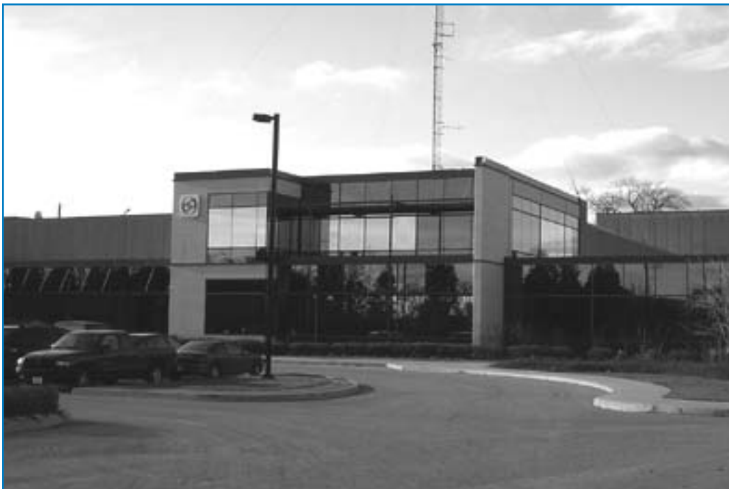
PHOTOS COURTESY SELECTPOWER INC.
