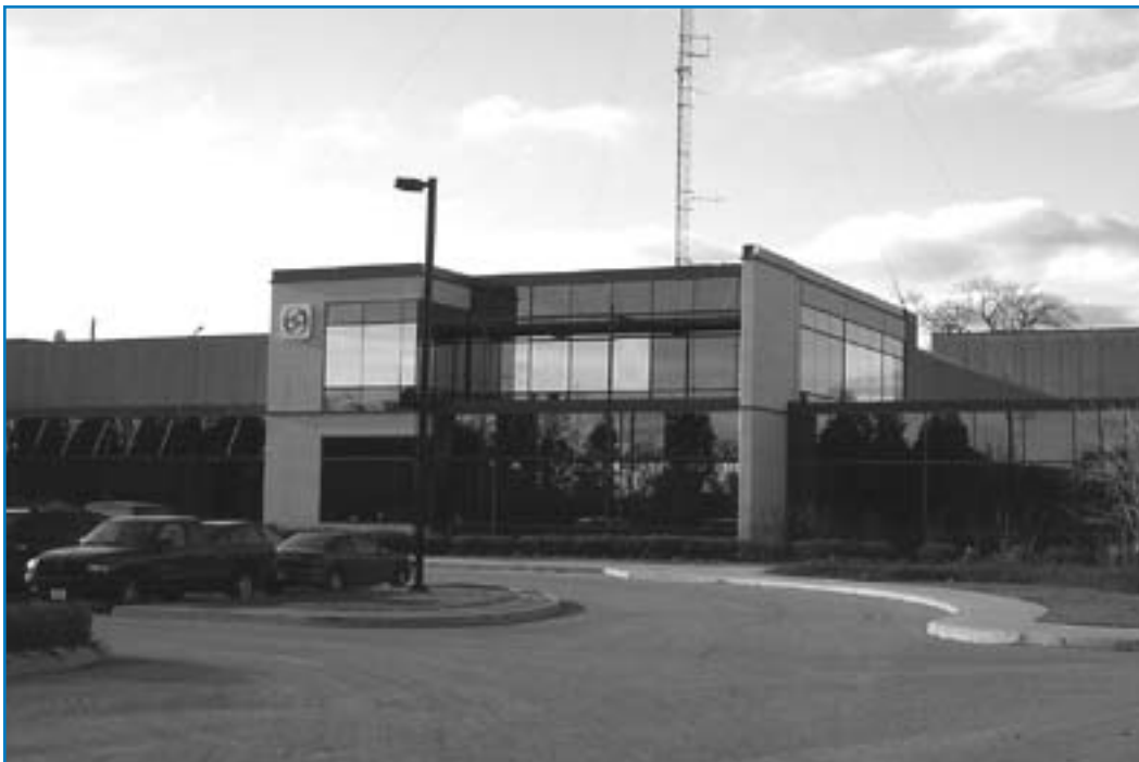
PHOTOS COURTESY SELECTPOWER INC.
