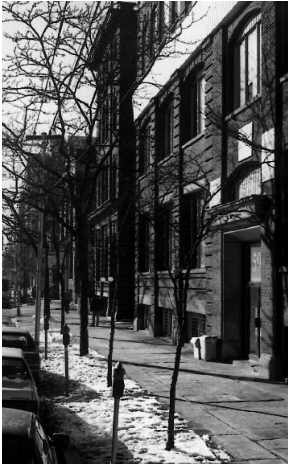
Looking along King Street west of Spadina Ave.
