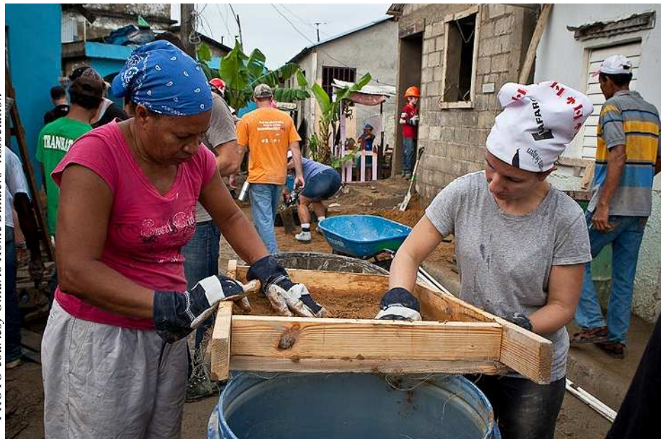
PHOTO courtesy Ontario Home Builders' Association
